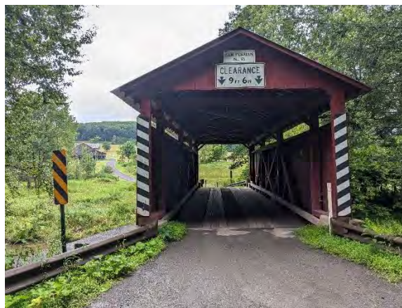
Kramer Bridge over Mud Run in Greenwood Township, Columbia County
